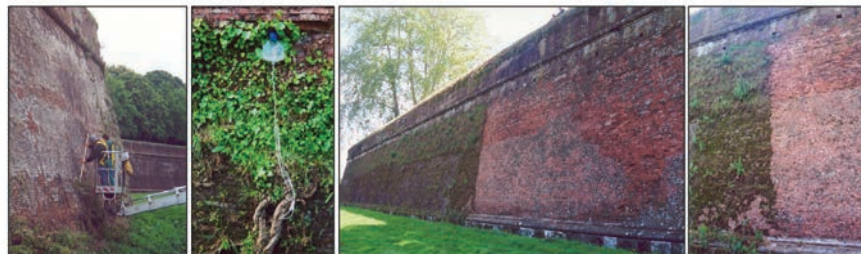
Figura 5. Lucca Walls. Step 2 (mechanical interventions); Step 3 (herbicide injection in Hedera); Step 4 (treatment effect with herbicides). (Photo Bertoncini-Lorenzoni, Lucca 2001).
