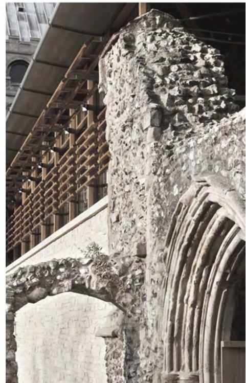
Fig. 11-12: Cittadella Walls, Padua, Italy. Project by Patrizia Valle (1994-2013). Reconstructed patrol walkway Porta Padova. The restoration focused primarily on maintaining the city walls, using materials and building techniques compatible with traditional ones (ph. Andrea Pizzato).
