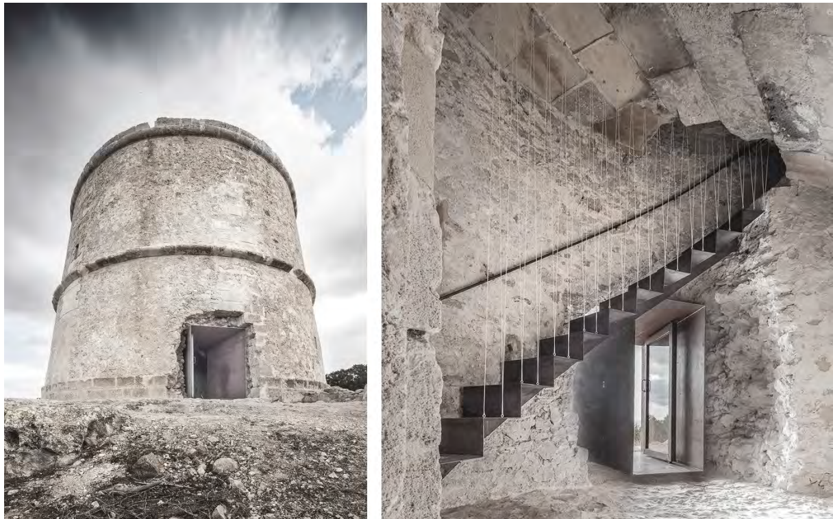
Fig.10-11: Pi des Català tower in Formentera, Spain. Project by Marià Castelló Martínez (2009-2015). View of the entrance and detail of the steel staircase (ph. Marià Castelló).
