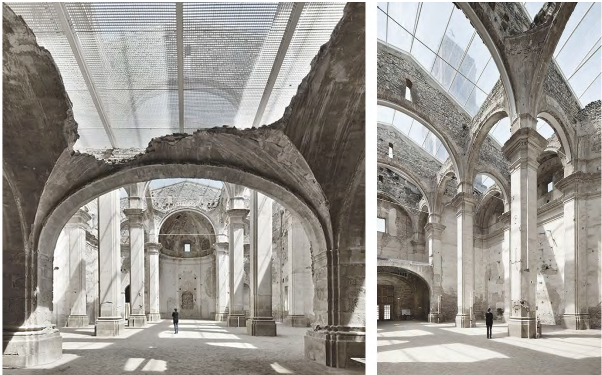
Fig. 6-7: Church of san Pedro, Corbera d'Ebre, Tarragona, Spain. Project by Ferran Vizoso (1999-2011). Views of the large skylight in transparent and light panels (ph. Jose Hevia).
