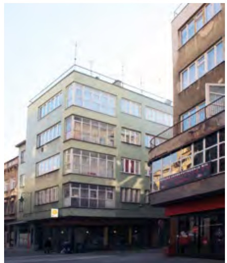
Reuf Kadić, Buildings on Ferhadija Street (1939-1946)
