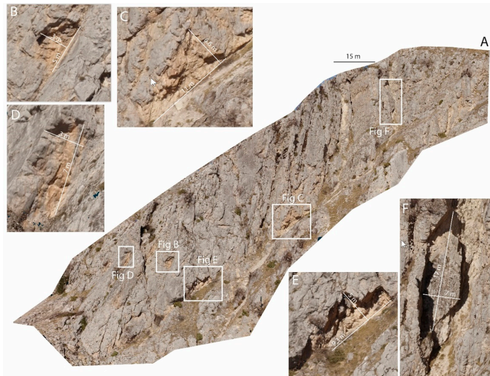
Figure 17. The 3D model of the area UAV 2 (A), examples of rockfall scars (B–E) and a suspended block (F). The calculated volume of failed blocks associated with such scars is ca. 40 \text{ m}^3 (Figure 17B), ca. 200 \text{ m}^3 (Figure 17C), ca. 60 \text{ m}^3 (Figure 17D) and ca. 230 \text{ m}^3 (Figure 17E). Figure 17F highlights the volume of overhanging block with a volume of ca. 500 \text{ m}^3 .
