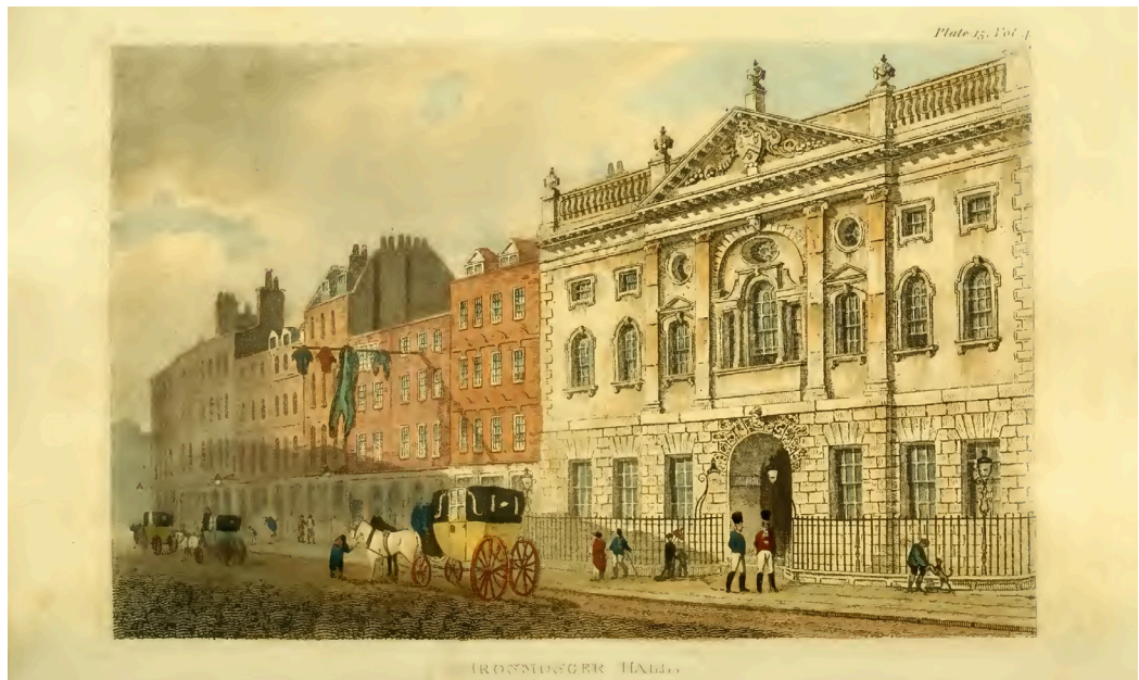
Fig. 01. Ironmongers' Hall (The Repository of Arts, March 1811, plate 15).
