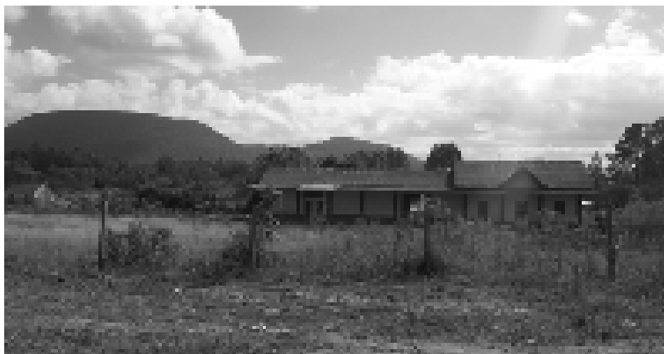
Figure 3. Abandonment of the building and surroundings of the old railway station of Camobi. Source: Paula Polli.
