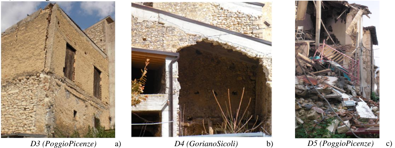
Fig. 7. Out-of-Plane overturning in absence of iron ties associated to damage levels of (a) D_3 , (b) D_4 and (c) D_5
