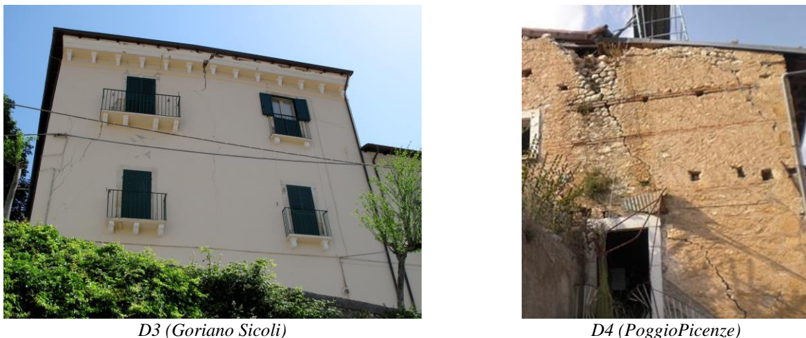
Fig. 8. (a) Flexural and (b) overturning with side wing of two facades
