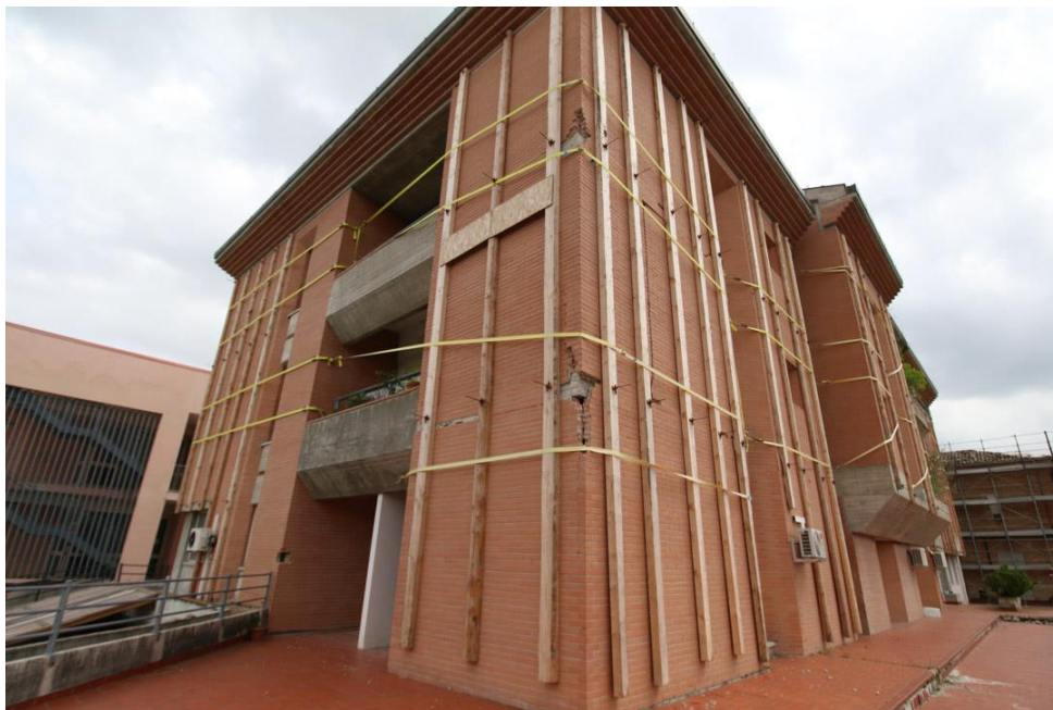
Fig. 2.5 – Separation of the external brick coating and provisional supports.
