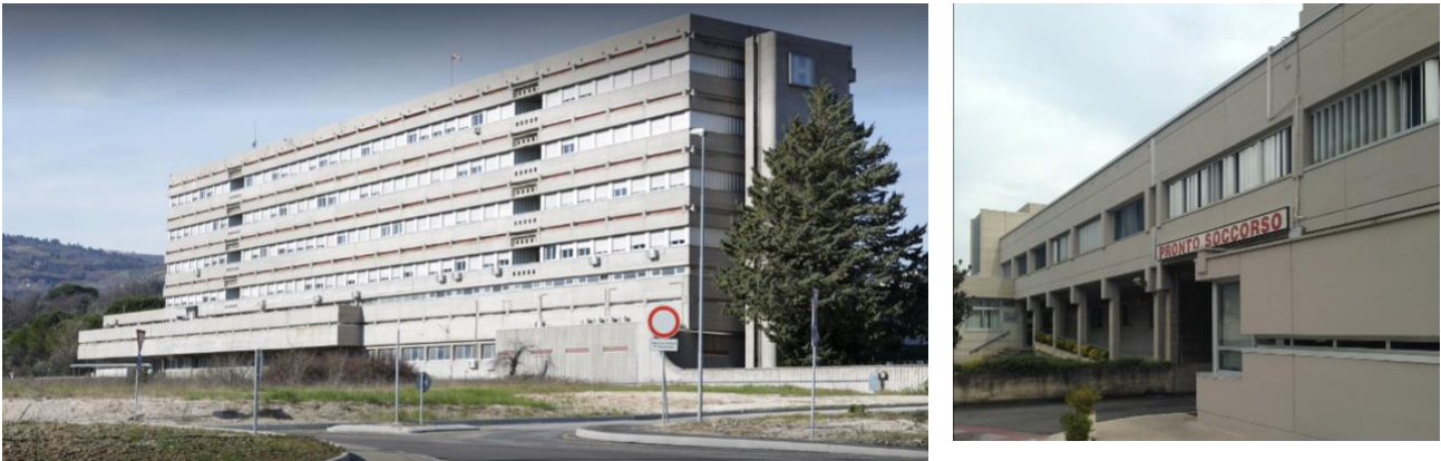
Figure 4.2.3. – Global frontal view (left) and main entrance of the Emergency Unit (right) of the San Bartolomeo Eustachio Hospital, San Severino Marche, Macerata.
