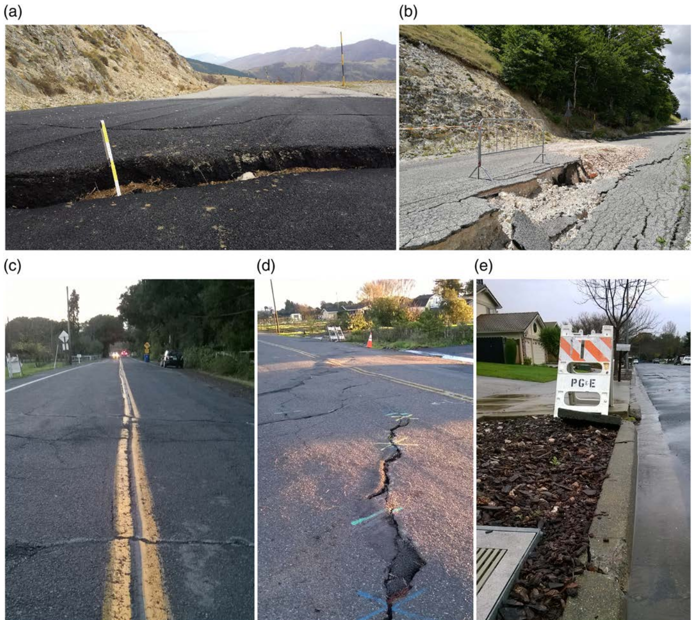
▲ Figure 1. Surface ruptures related to moderate earthquakes, either on the principal or distributed (synthetic or antithetic) faults, can lead to significant damage to infrastructures and lifelines. (a,b) Surface faulting during the M_w 6.5 Norcia earthquake (30 October 2016) affected mountain roads and temporarily impeded traffic, both along (a) principal and (b) secondary antithetic segments (pictures in November 2016 and July 2017, respectively). (a) The fault offsets the new asphalt that was set up after a first damage to the road during the 24 August 2016 M_w 6 foreshock. (c–e) The roads crossing the principal fault strand that ruptured during the M_w 6 West Napa earthquake (24 August 2014) were severely damaged by (c) parallel or (d) en- é chelon segments, and several tiny (several centimeters) dextral offsets even damaged installations (curb and buried Pacific Gas and Electric Company pipes) crossing (e) secondary segments (pictures in December 2014). Note that panel (d) additionally illustrates the occurrence of postearthquake aseismic slip (afterslip) with the shift of the paint marks. The color version of this figure is available only in the electronic edition.
