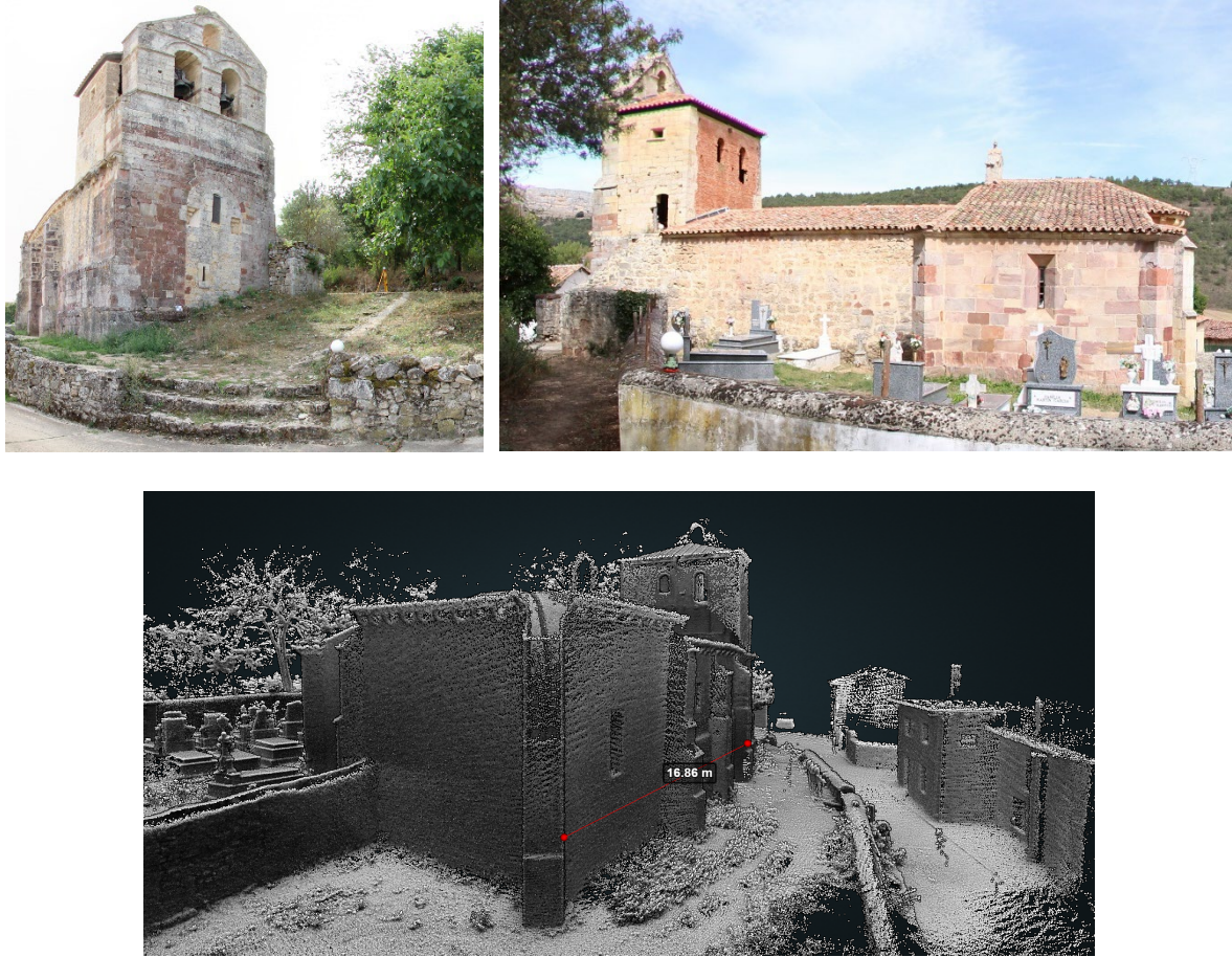
Figure 7. Church of San Pedro: exterior views (top) and representative perspective from the final point cloud (bottom).
