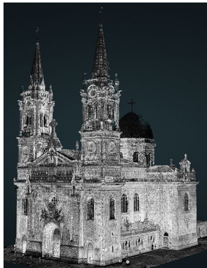
Figure 5. Church of São Torcato: exterior view (top) and representative perspectives from the final point cloud (bottom).
