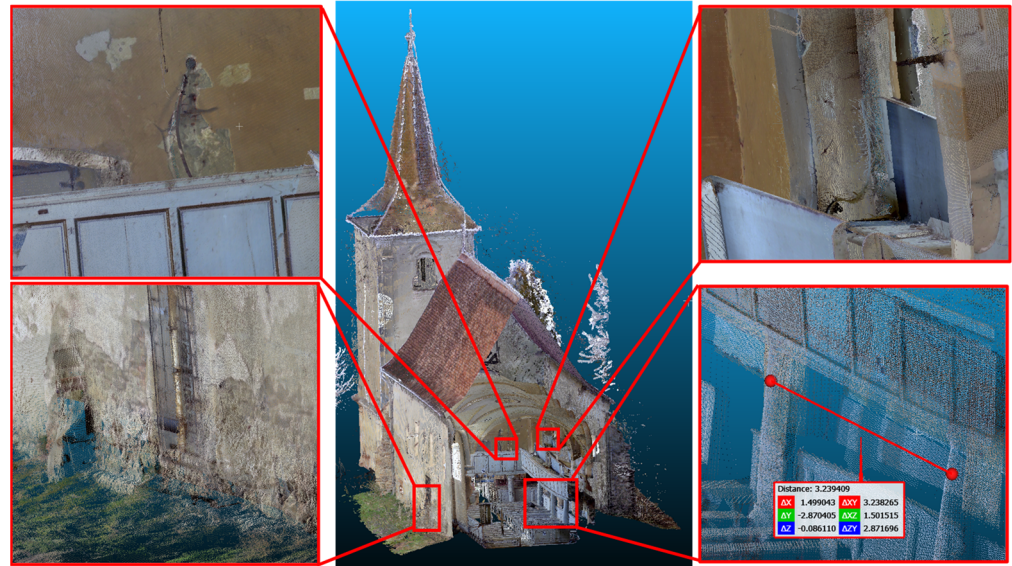
Figure 6. Existing condition modeling for current condition assessment and structural measurements.
