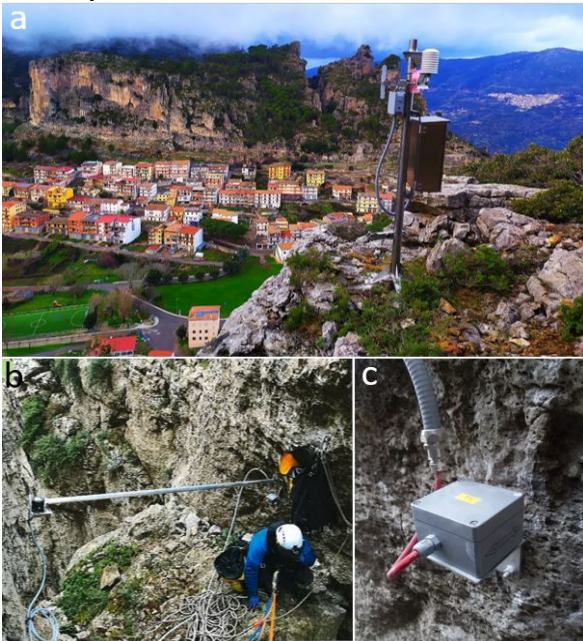
7 – Geotechnical station trumentations a) Data logger station 1 on Tisiddu Mountain; b) Extensimeter Ext 1; c) Tiltmeter Tilt1.
