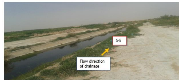
Figure 3 Good functioning of drainage ditches (oasis 2). There is no risk of degradation of the palm groves.
