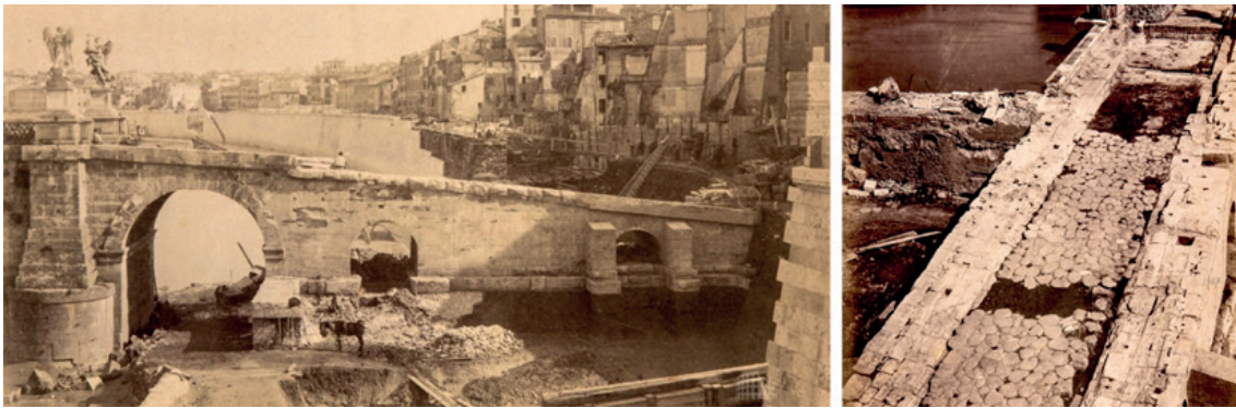
Figure 15. The ramp of Pons Aelius (Ponte S. Angelo) being demolished during the construction works for the Tevere's embankment, 1890 ca.
