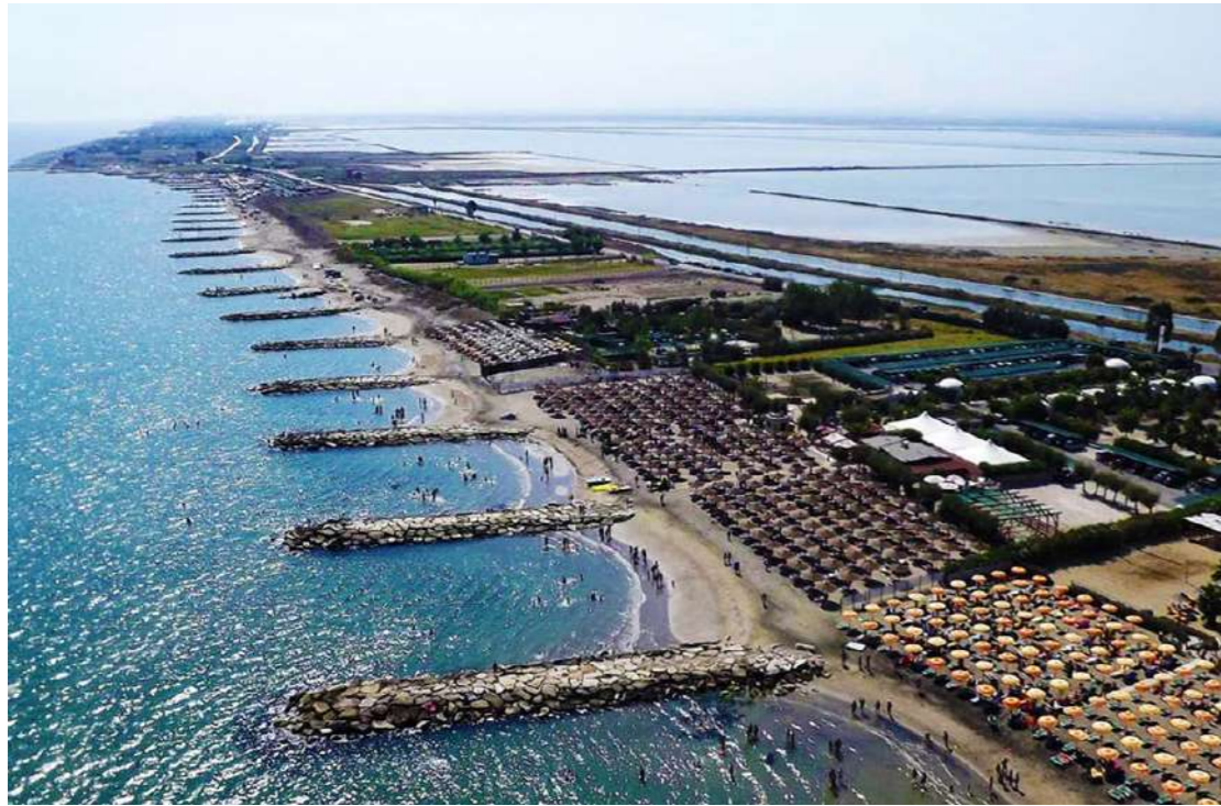
Fig. 02_ Groins to counteract coastal erosion in the northern coastline of Margherita di Savoia. Photo by BATmagazine, https://www.batmagazine.it/ , 2021
