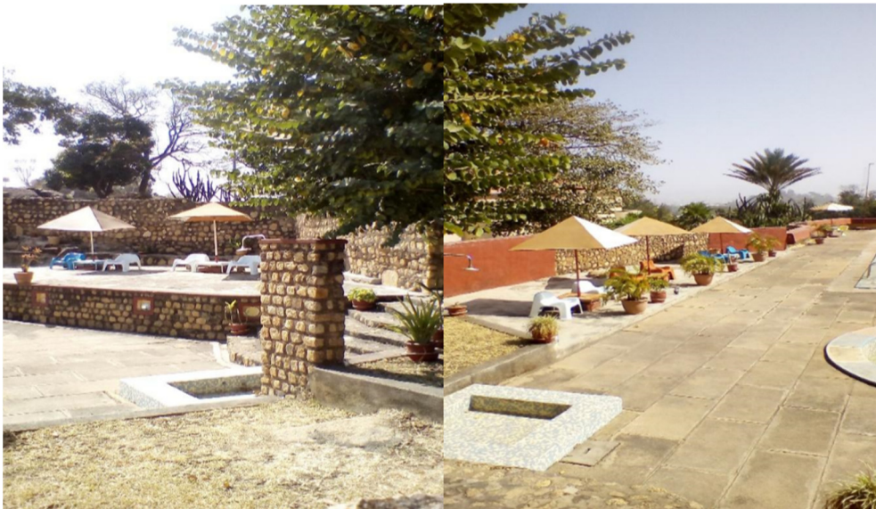
Figure 8: Perfectly cut flagstone from limestone used for wall caps, pool decks, garden walkways, and patios [23].
