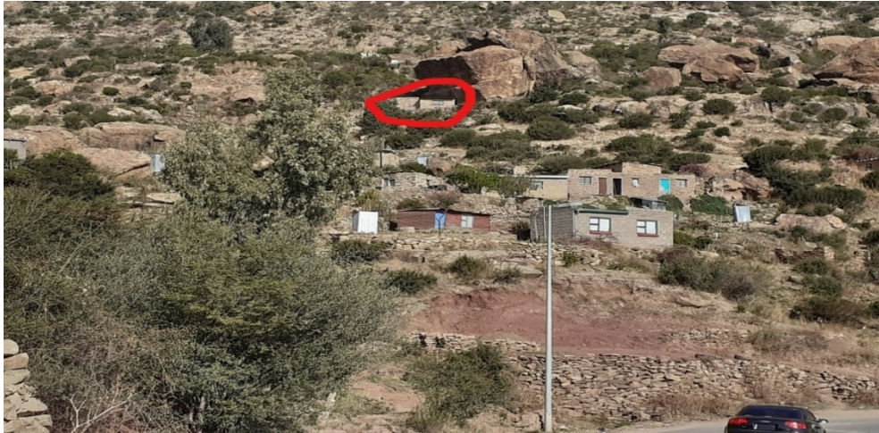
Figure 1: Settlements susceptible to rockfall in Maseru. (Source: Authors Field Survey, 2022.)
