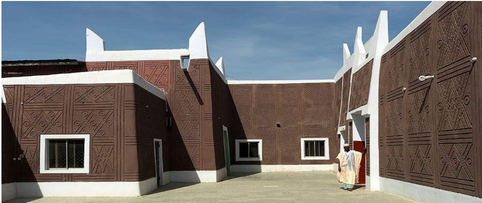
Figure 5: Adobe used as a building material in constructing the 15th-century Gidan Rumfa in Kano [14].
