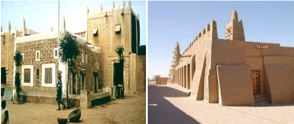
Figure 6: Adobe used as building material [10].
