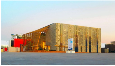
Figure 4: BIPV ventilated façade at BX house. Figure 5: BIPV window at VT house's foyer. (Source: SDME Organization.)
