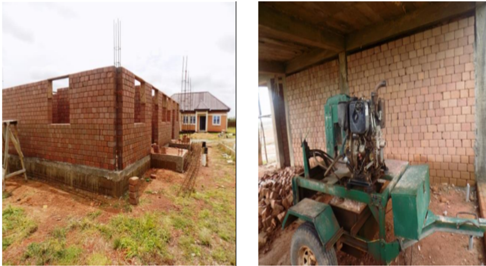
Figure 10: A house under construction using NBRRI CEB technology in north-central Nigeria.
