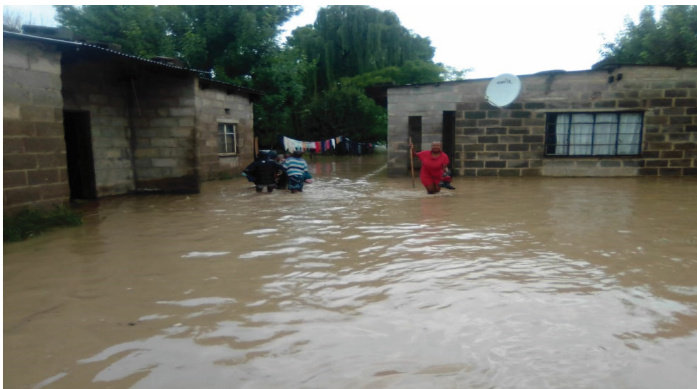
Figure 2: Flooded houses in Maseru in January 2022 [20].
