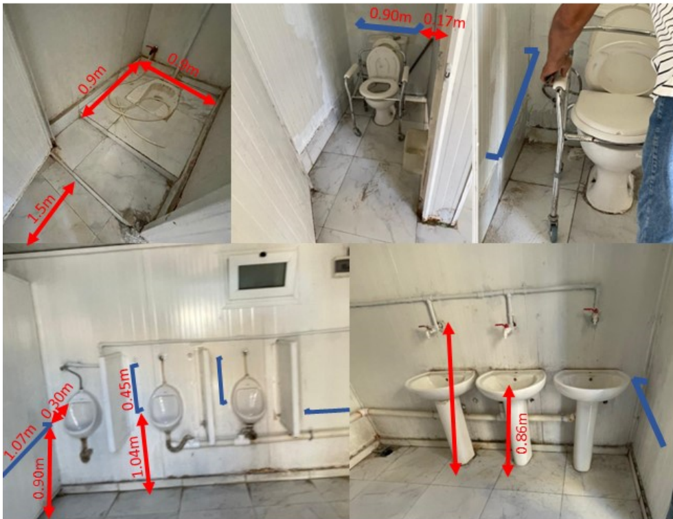
Figure 10: Accessible toilet suggestions at building A.
