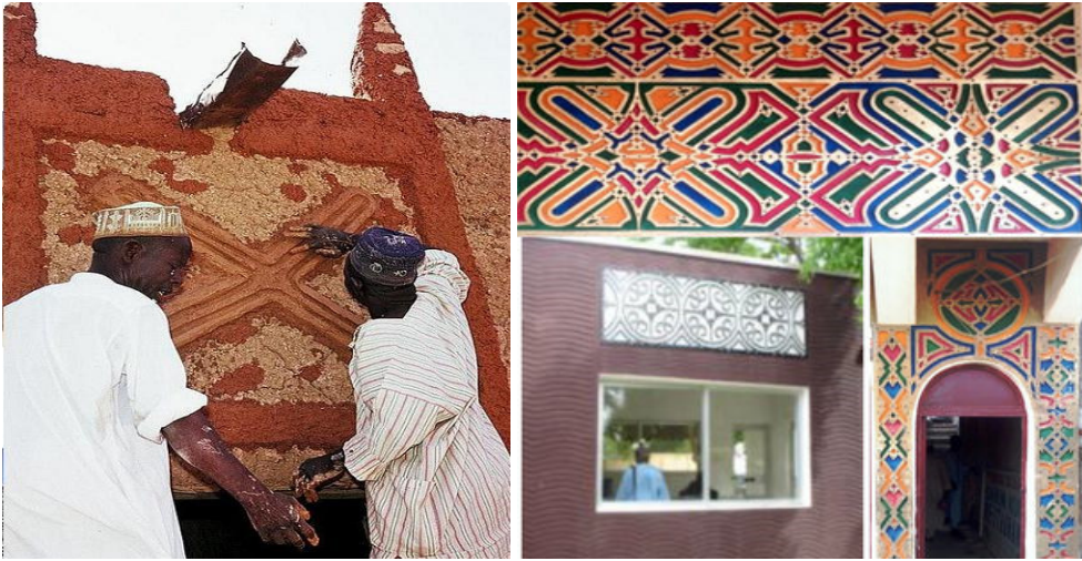
Figure 9: Engraving works on the façade [14].
