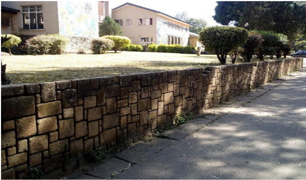
Figure 7: Stones used as retaining wall [23].
