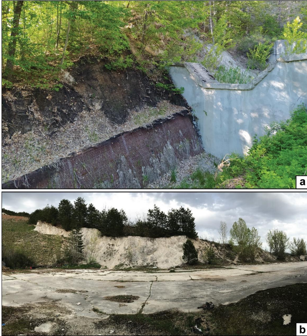
Figure 4.14. Main anthropic landforms detected in the study area. a) Solid transport control system consisting of check dams and artificial channels; b) Cataclastic rock quarry located at the slope toe.
