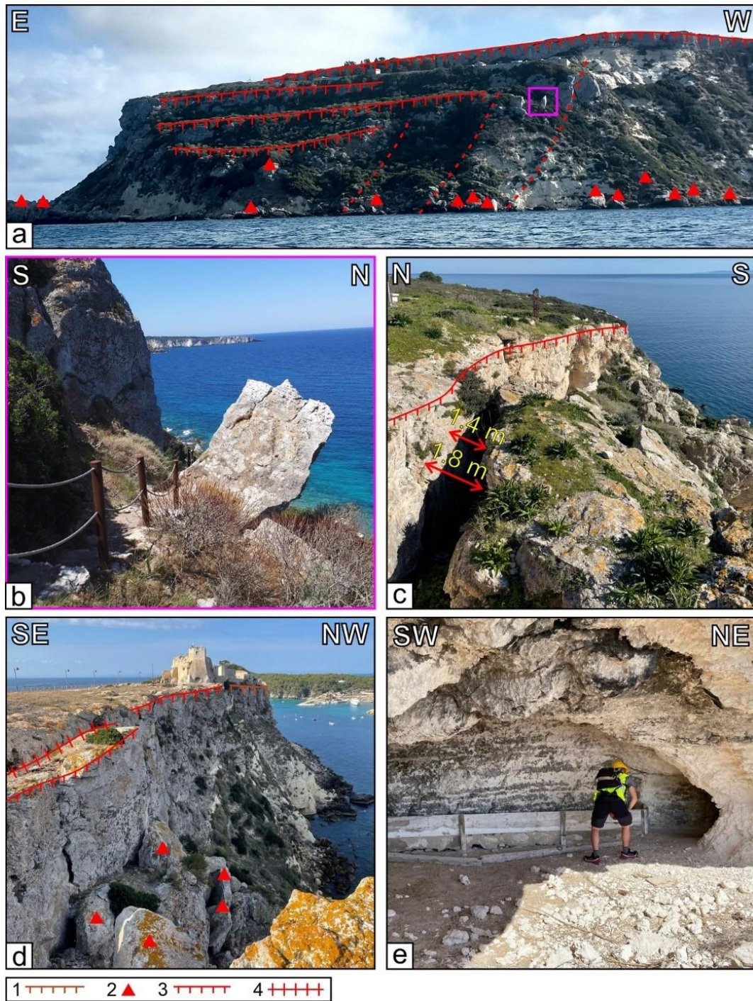
Figure 5.6. Photo documentation of geomorphological features of San Nicola Island: (a) landslide scarps, inferred sliding surfaces, and meter-sized fallen block detected in correspondence of Punta del Cimitero; (b) unstable meter-sized block of dolomitic limestone lithology detected in the Cemetery area—the position is indicated by the violet polygon in Figure (a); (c,d) deep trenches and rockfall deposits along the southern flank, east of la Tagliata, and the northwestern one of Pianoro di San Nicola; (e) anthropic cave carved into marly deposits. Legend: (1) structural scarp, (2) isolated block, (3) slope scarp, (4) trench.
