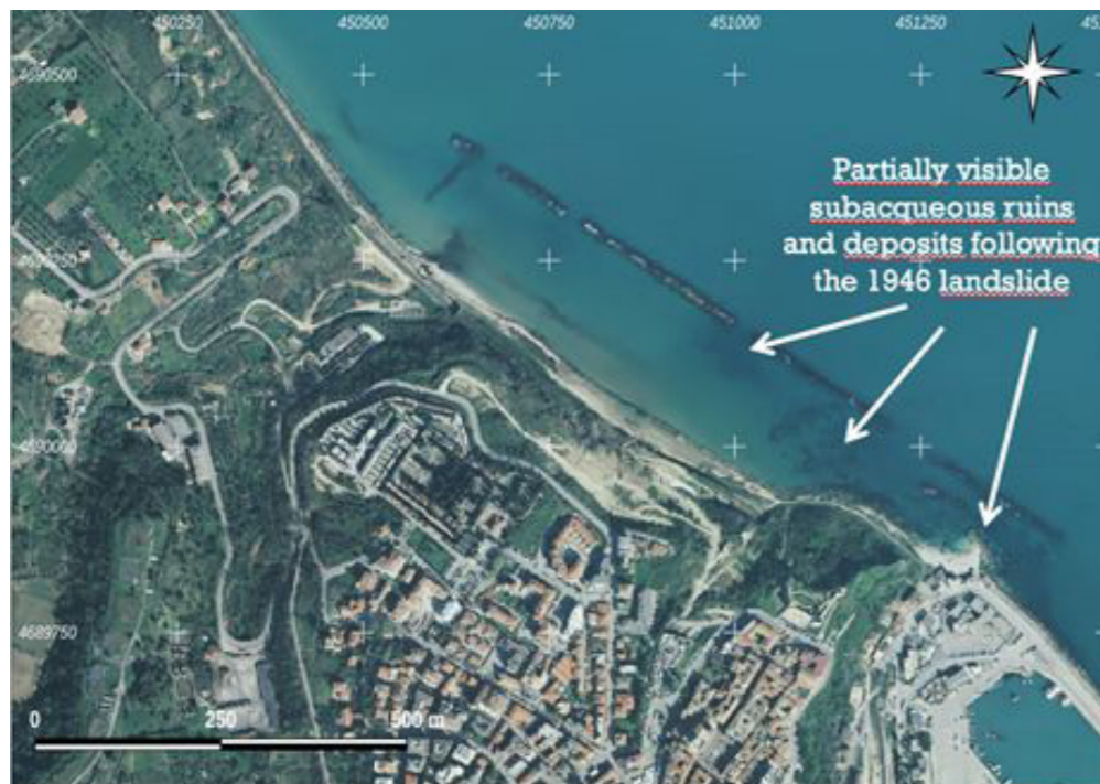
Figure 17. Aerial image 18 of the Ortona coastline in the 'Lo Scalò' site, in the northern side of the modern harbor, where subaqueous landslide deposits and ruins are visible.
