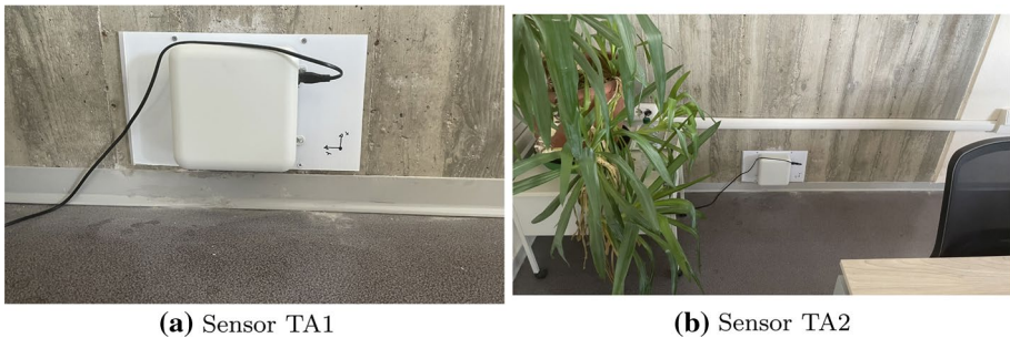
Fig. 9 Deployed sensors for the fourth elevation of C2 building
