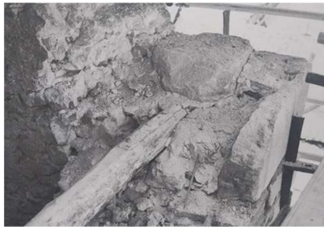
Figure 11. Wooden element inside the masonry of S. Biagio D’Amiterno in L’Aquila (source: [69]).
