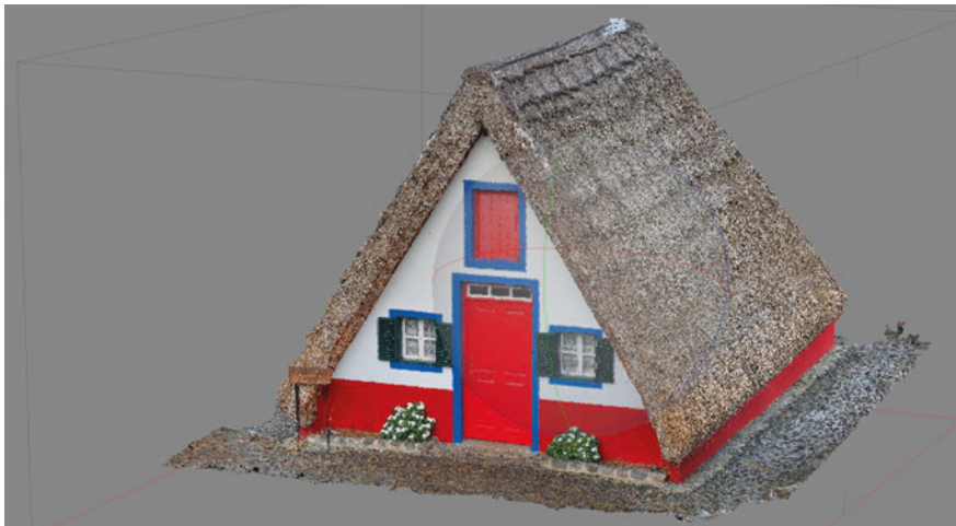
Fig. 6 A lightweight textured mesh generated from the digital photogrammetric survey of the traditional San Sebastian House (Madeira, Portugal) (Editing: Authors in 2022)
