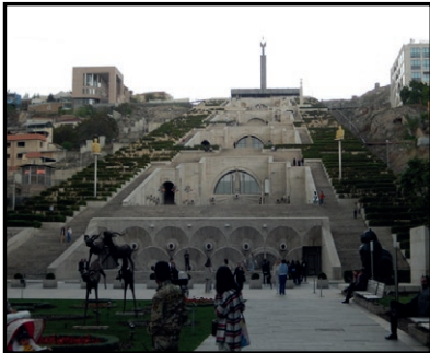
Bottom view of the Cascade complex from the Tamanyan Street
