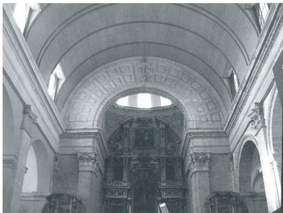
Fig. 2. Medina Rioseco, Valladolid. Santa Cruz church. The laminated wood in the nave characterized the interior space (Verazzo 2007).
