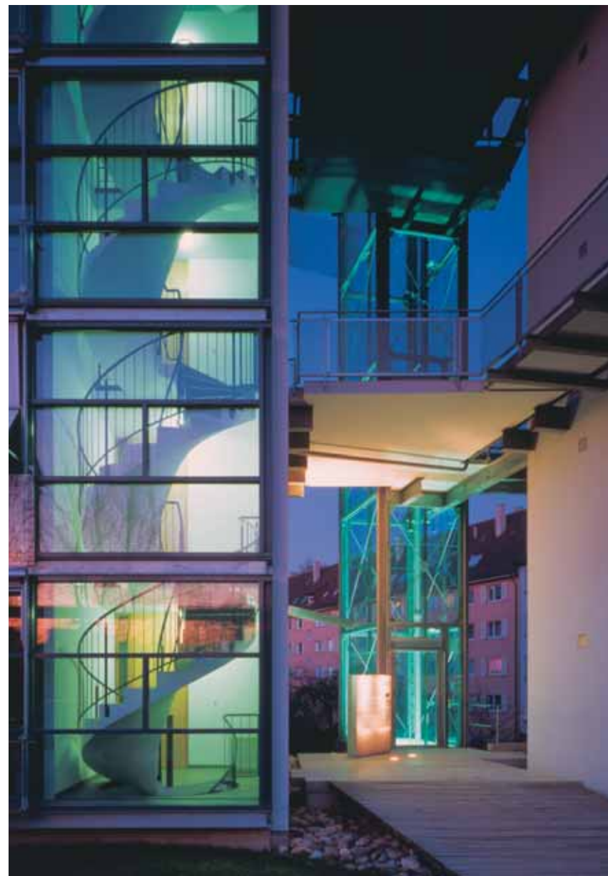
Erick van Egeraat/Mecanoo, Edifici residenziali a Stoccarda, 1993. Il sistema distributivo Erick van Egeraat/Mecanoo, Residential buildings in Stuttgart, 1993. The system of
