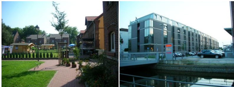
Figure 8 . The neighborhoods of Marxloh, Innenhafen (Social Housing). Foster + Partners for Duisburg.
