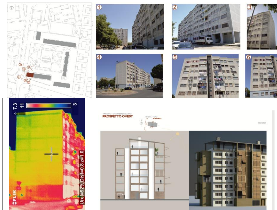
Figure 6 . Photos of the residential complex. Thermo graphic measurement and hypothesis of project of transformation
