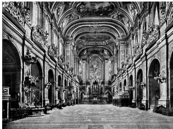
Fig. 03 - Napoli, internal view of the Santa Chiara's church before the Allied bombing of 1943, photographic archive of the Superintendence for Architectural Heritage for Naples and its province (ASBAN).
