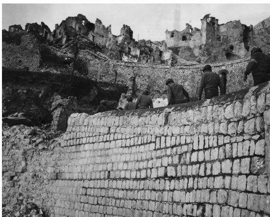
Fig 11 - San Pietro Infine (CE), buildings destroyed after December 1943 (Maslowski 1993)
