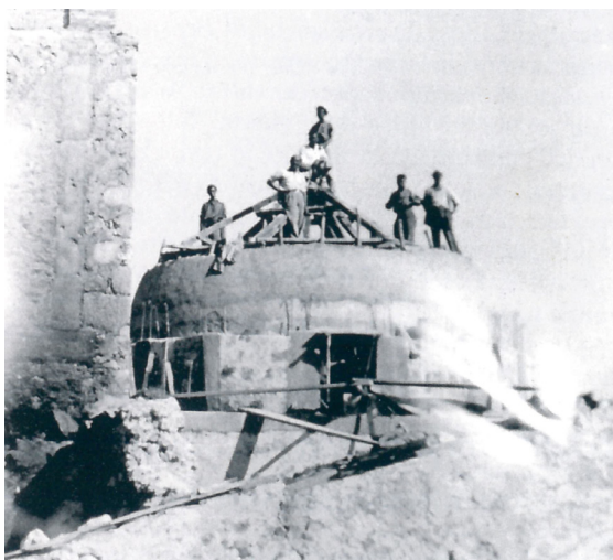
Fig. 02 - San Pietro Infine (CE), the post-war reconstruction of the dome of San Michele Arcangelo with the use of reinforced concrete (Zambardi 2003)
