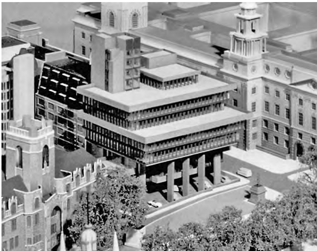
7. Denys Lasdun, Royal Institution of Chartered Surveyors (RICS) a Parliament Square, Londra, 1963. Veduta del modello.
