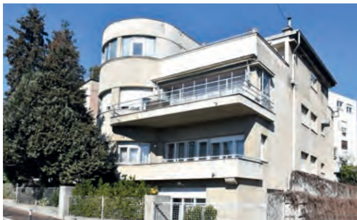
20c. In alto a sinistra: M. Kaulzarić e S. Gomboš, Villa Spitzer, veduta d'epoca, via Novakova. Zagabria, 1930-31. Da E. Blau, I. Rupnik, Project Zagreb. Transition as Condition, Strategy, Practice
