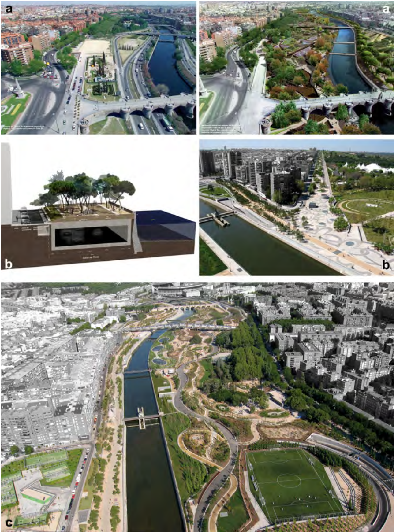
(Fig. 7) Parque Río Manzanares , Madrid. Project: by West 8 + Burgos & Garrido + Porras & La Casta + Rubio & Álvarez-Sala. 7a. The project area before and after the interventions; 7b. Cross-section along the M-30 highway with Salón de Pinos park areas and connection with the Avenida de Portugal ; 7c. Aerial view on Arganzuela Park areas.
