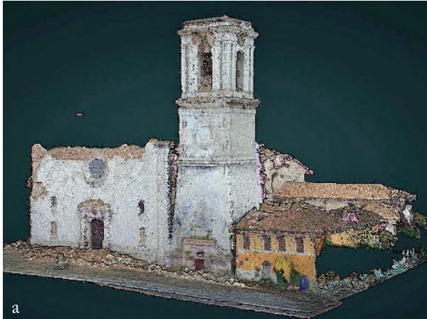
Fig. 3. Norcia, cathedral of S. Maria Argentea. Post-earthquake laser scan survey (2017).
