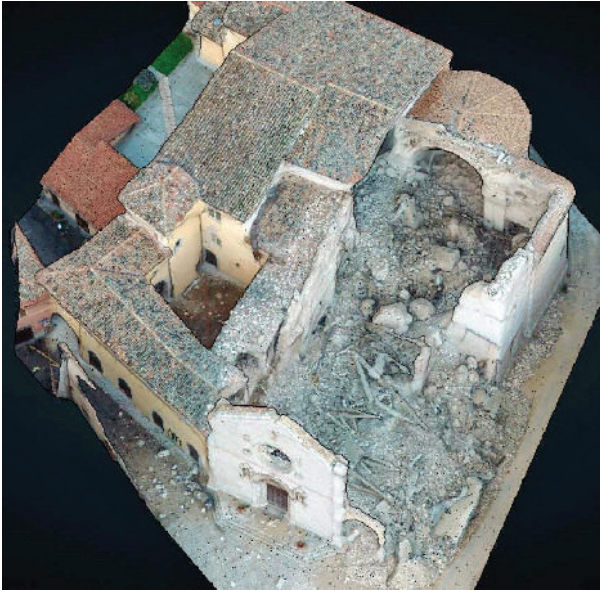
Fig. 4. Norcia, S. Benedetto. Laser scan survey after the earthquake of 30 October 2016.
