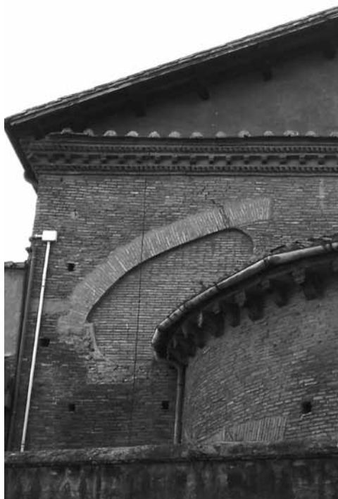
Fig. 11 - Rome, basilica of Santa Cecilia in Trastevere, an eighteenth-century opening round the apse created to enhance lighting of the nave (later closed during restorations; photo Author).
