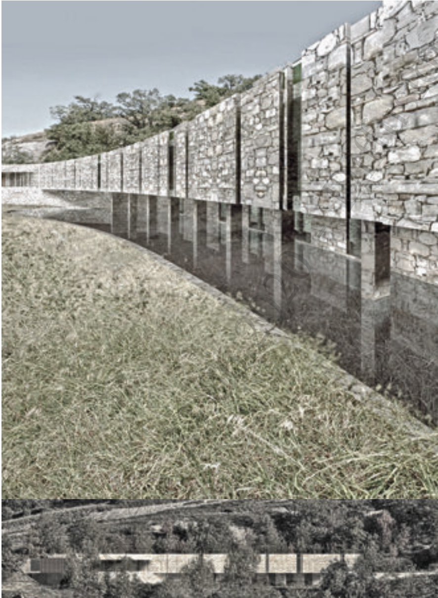
Figures 10-11: The Dwelling Wall: New Volumes as centre for research, knowledge, and culture of the whole territory.
