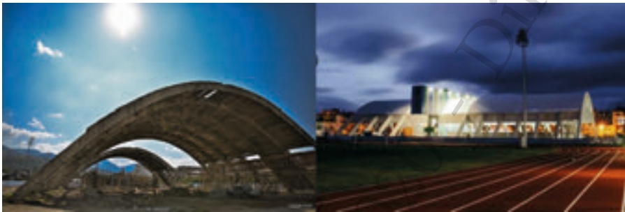
Figure 13: "The Multifunctional Children's Centre" the structure where the new building is based. Source: Municipality Archive
