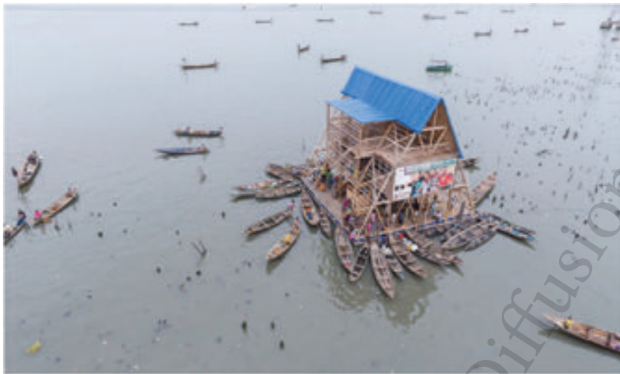
Figure 4: Floating School, Makoko Lagos (Nigeria), Kunlé Adeyemi 2012
