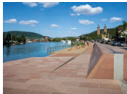
Figure 6: The "additive wall" to defend against flooding. Photo by Harmut Holl
