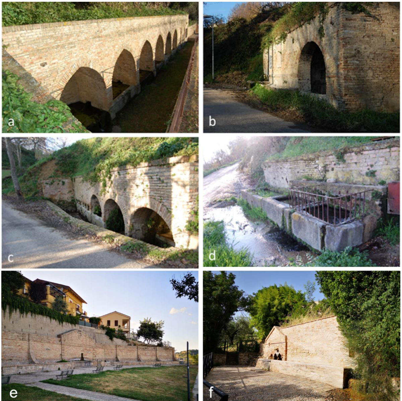
Figure 3. Some examples of tapped springs of the study area discharging at the interface between permeable and non-permeable lithotypes located at the border of the historical town of Atri (a–d), Chieti (e), and Pescara (f); (a,e,f) are examples of architectural restoration.
