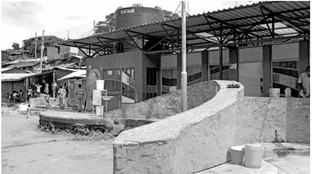
One of the spaces built by KDI in Lindi village provides water and sanitation facilities in addition to communal gathering space and play areas.
