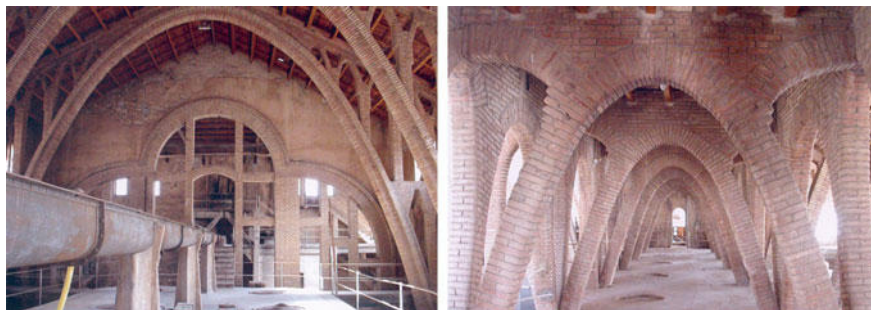
Fig. 3 Pinell de Brai: internal views of the vaulted systems
