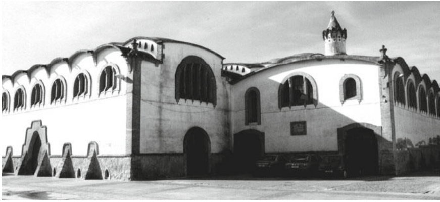
Fig. 13 Gandesa: external view main front facade
