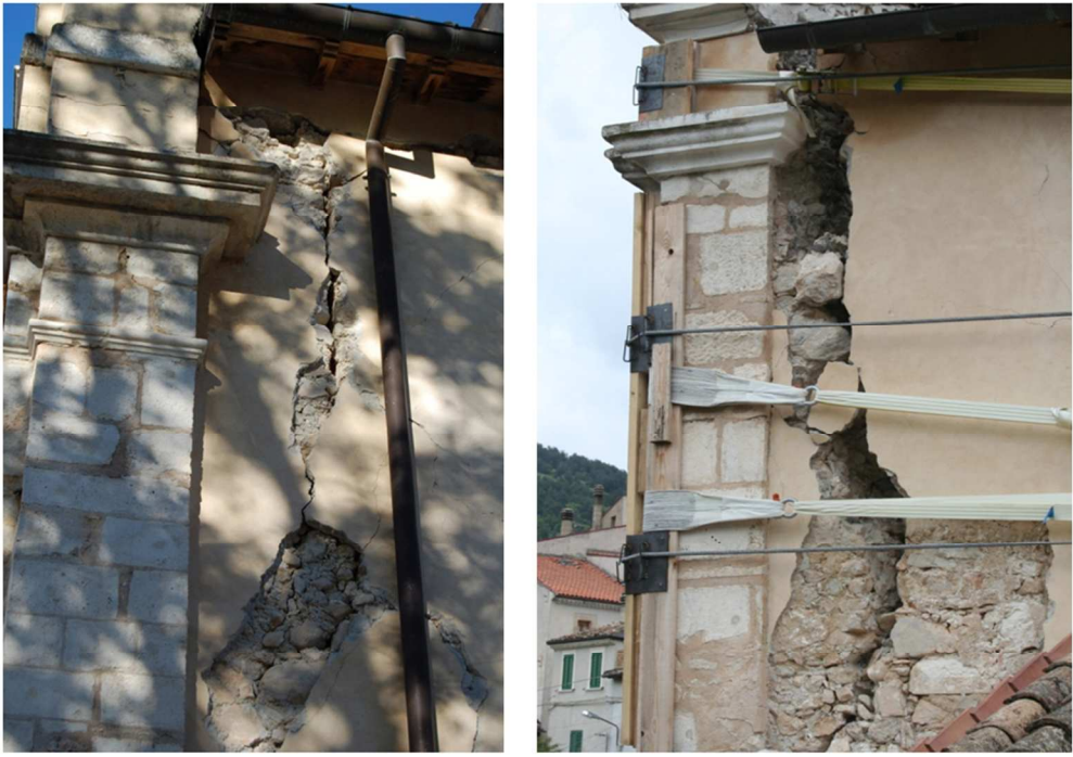
Figure 16. Façade overturning in St. Gemma church (SGM) in Goriano Sicoli. 83x58mm (300 x 300 DPI)
