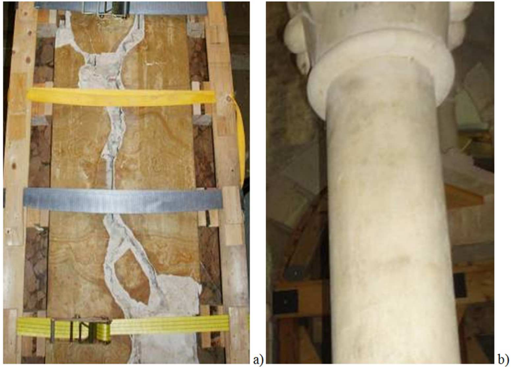
Figure 14. Observed damages after the 2009 seismic event on a) rubble masonry pillars of St. Gemma church (SGM) in Goriano Sicoli; b) not damaged monolithic columns in St. Pietro ad Oratorium (SPO) in Capestrano.
