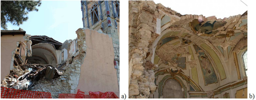
Figure 22. Collapse of the a) St. Nicandro e Marciano Church (SNM) in L'Aquila (Roio Piano) and b) St. Gregorio Magno Church (SGO) in L'Aquila (San Gregorio) after the 2009 seismic event. 85x33mm (300 x 300 DPI)
