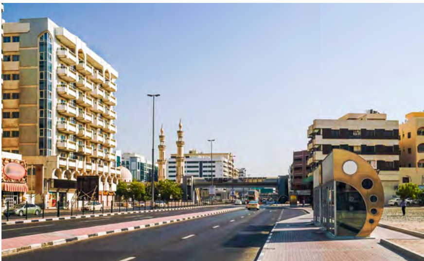
Fig. 3 - Air-conditioned bus-stops in the district of Al-Rigga: an example of the use of air treatment systems also in the outdoor spaces due to high temperatures (Stanistav Sablin, 2020).
